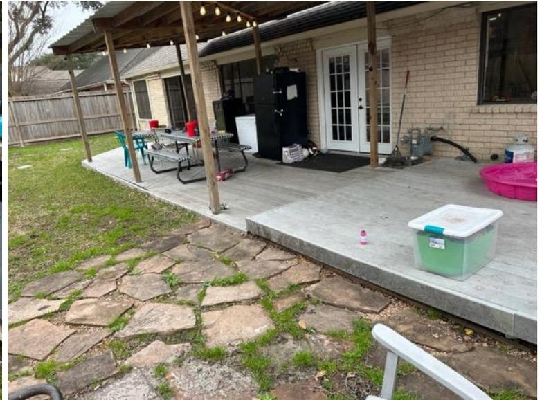
Wood to ground contact – Deck should be monitored for insect activity.
