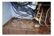
$\ensuremath{\boxtimes}$  Debris/rust observed at the interior of the service equipment disconnecting means panel board enclosure.
