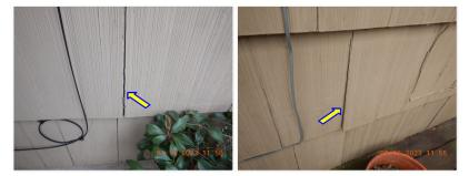
☑ Caulking is needed at all joints and unsealed seams in the siding.
