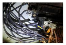
☑ The black insulated conductor used for grounding and or bonding should be marked green.
