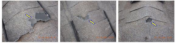
☑ Missing or damaged ridge cap shingles were noted. ROOF JACKS/VENTS:
