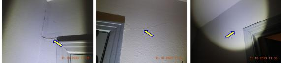
☑ Cracks/damage/repairs in the drywall observed.
