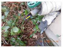
☑ Exterior hose bibs not installed with anti-siphon devices at some locations.
