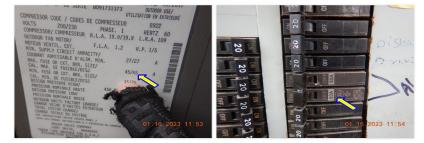
☑ Circuit breaker installed at A/C condensing unit circuit is too large per manufactures specifications. 50 amp installed and 45 amp is required per manufactures specifications.
