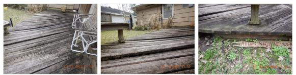
$\square$  Deteriorated wood decking boards from weathering at the back patio. Several of them are raised and are a trip hazard.
