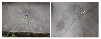
Settlement cracks observed at the flatwork at the following locations: Front walkway, Driveway.
