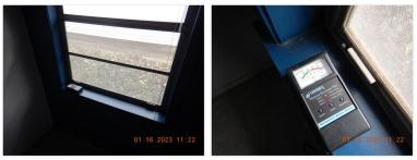
☑ Window area- Higher than normal (Relative reading of 14 -- 19) moisture readings were noted with the moisture meter in the tested area.
