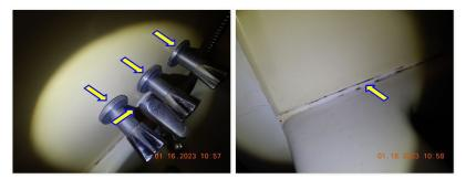
☑ Caulk the bathtub/shower enclosures and around fixtures where missing or deteriorated. COMMODE:
