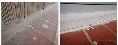
$\square$  Caulking is deteriorated where the siding butts up against the brick. FLASHING
