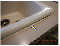
☑ Caulk missing or deteriorated around the sink rims at the following locations: Kitchen. <u>TUBS/SHOWERS:</u>
