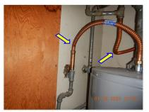
$\square$  Hot and cold water lines should be insulated within 5' of the unit. DRAIN PAN:
