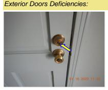
$\square$  All exterior door locks should be keyless operation from the interior was noted. Some Examples: Front door. The deadbolt could not be unlocked at the time of inspection.
