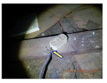
$\blacksquare$  Exposed wiring and an older 2 prong plug was noted in the attic.
