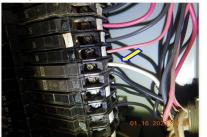
☑ The white wire connected to the 240 volt circuit breakers should be marked with a color (red or black).
