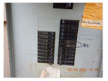
$\boxdot$  Branch circuit service locations were not all marked at the service equipment disconnecting means panel board enclosure dead front cover.
