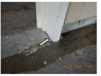
$\ensuremath{\boxtimes}$  Garage door jambs in contact with the slab surface and are not chamfer cut.
