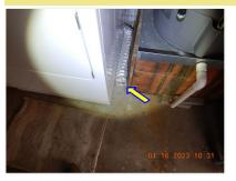
Dryer vent pipe is disconnected and/or discharging into the garage.
