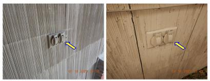
☑ Exterior receptacles are currently required to have a "weatherproof while in use" cover, also known as a plastic "bubble cover" type.
