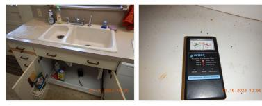
$\square$  Sink cabinet area- High moisture readings were noted with the moisture meter in the tested area.
