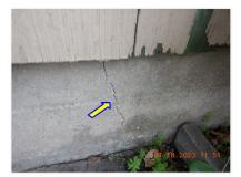
☑ Cracks observed at the slab perimeter.
