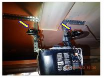
$\square$  Photoelectric sensors are not properly installed at the base of the garage door. The sensors should not be installed more than 6 inches above the garage floor.
