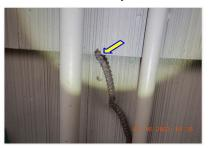
☑ Grounding conductor clamp at the grounding electrode is loose or is disconnected.
