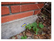
☑ Corner fractures (possible insect penetration) SLAB CRACKS:
