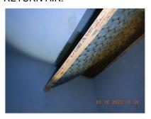
$\square$  No return air frame is in place in the front right bedroom closet. A filter has been jammed in place at this location.
