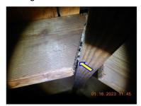
☑ Rafters cuts not flush at the ridge, hip and or valley boards in the attic.
