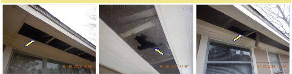
☑ Soffit area screens are missing and/or damaged at multiple locations. *Attic Framing Deficiencies:*
