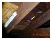
☑ Roof covering wood supports are damaged at some locations. *Attic Moisture Deficiencies:*
