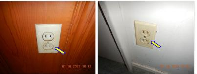
☑ Older 2 prong plugs are in use at multiple locations. These are an older style plug that are not grounded. These types of plugs were used prior to the 1960s.
