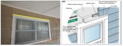
$\square$  The window and/or door and/or other wall penetrations installed through the wood fiber products siding were not properly flashed.
