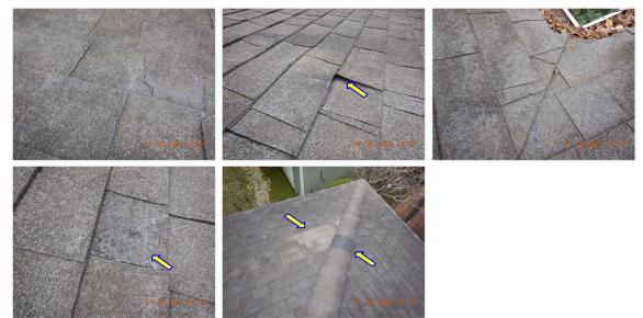
☑ Scuffed and/or damaged shingles were noted. Possible repairs were noted at some locations.
