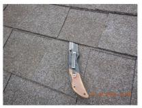
☑ Per the Texas Real Estate Commission Standard of Practice effective February 1, 2009, home inspectors are required to inspect shingle fasteners. To inspect fasteners, the lower tab of the shingle must be lifted at several locations. As is the case in most homes, this inspection was not possible without damaging the shingles. Under the Standards of Practice departure clause this item was not inspected.
