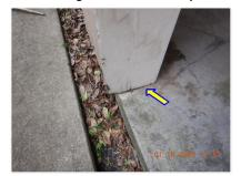
$\square$  Siding is in direct contact with the flat work. Water that accumulates at this area can cause the siding to rot/deteriorate.
