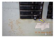
☑ Note: One of the circuit breakers was tripped at the time of inspection. This could possibly be the cause for some lights and/or plugs having no power at the time of inspection.
