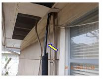
$\ensuremath{\boxtimes}$  Insulation is missing or deteriorated on the A/C suction line at the condensing unit.
