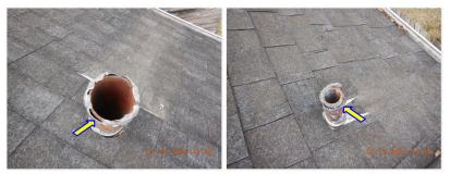
☑ Lead coverings at the roof jacks is damaged/deteriorated.
