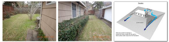
The drainage and grading around this home is inadequate. In order for the drainage to be effective, the landscaping must be configured so that the yard is sloped away from the foundation by at least 6 inches in the first 10 feet and/or adding additional gutters/downspouts to the house is another option to improve drainage and/or in- ground drains should be designed and added to divert rainwater and runoff away from the house as appropriate and/or drainage swale should be improved/installed.
