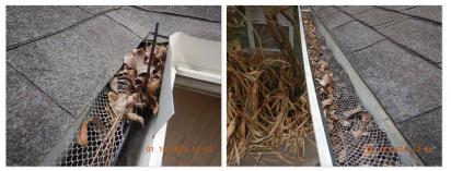
$\square$  Gutters should be cleaned frequently to prevent the accumulation of leaves and debris. Improperly secured gutters, as a result of weight from the accumulation, may cause potential damage to the adjacent exterior / soffits / fascia or roof.
