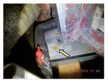
☑ Rust observed at the A/C auxiliary drain pan. Continue to monitor. INSULATION:
