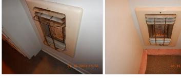
☑ Older wall gas heaters should not be used. These are considered unsafe.
