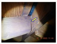
$\square$  Rafters were secured to the ridge board with 0 nails on one side, versus the appropriate number on one side, the appropriate number on the other.
