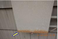
☑ The service equipment disconnecting means panel board dead front cover is rusted. INTERIOR PANEL BOARD:
