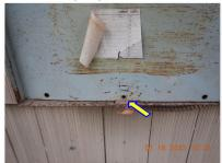
$\ensuremath{\boxdot}$  The service equipment disconnecting means panel board dead front cover is missing one or more set screws.
