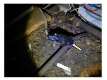
☑ Improper wiring splices observed, no junction box present, at the following locations: Attic. <u>WIRING AND CONDUIT:</u>
