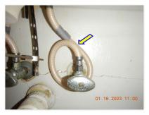
$\square$  Older vinyl style lines are in use at various plumbing fixtures. It is recommended that these be updated to the stainless steel type.
