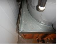
☑ Insulation/debris observed at the water heater auxiliary drain pan.
