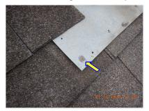
☑ Caulk face nailed roof jacks where missing. TREES:
