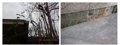
$\square$  The roof has tree limbs coming in close contact with the roof covering. Tree limbs can cause damage to the covering and allow access to the roof for unwanted pest. I recommend trimming back all tree limbs away from roof.
