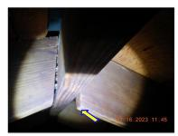
☑ Ridge boards are undersized. The ridge boards should be the depth of the rafter end cuts.
