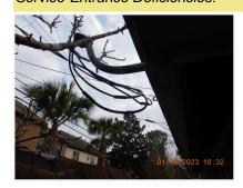
Service entrance wires do not have proper clearance from the ground and/or roof covering. Service Equipment Disconnecting Means Enclosure: General Electric Load Center Service Equipment Main Breaker Installed: 100 Amps
