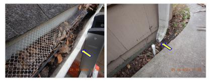
Dent gutters and directional diverters are damaged at some locations.
