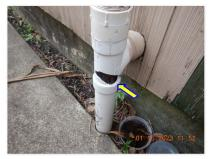
$\blacksquare$  Exterior plumbing clean out pipe is damaged at the left side of the home. SINKS:
