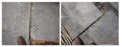
☑ The expansion joints in the driveway and walk way are open. Open expansion joints can allow water to get under the concrete surface and expand or wash away the soil causing lifting or settling of the concrete. I recommend filling the expansion joints with an approved expansion joint material.
