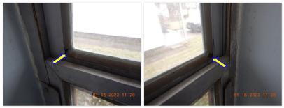
☑ Interior rubber window gaskets are separated at some locations. MOISTURE
