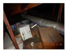
☑ The duct work at the attic is not strapped above the attic floor to prevent condensation from forming on the lines and dripping in the attic. RETURN AIR:
