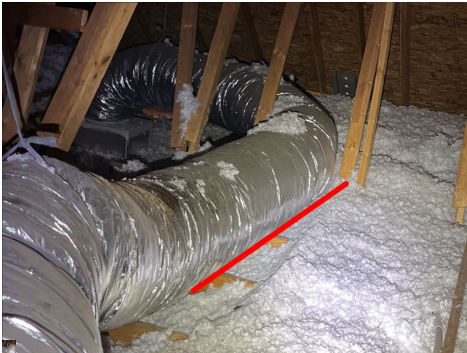
Duct on attic floor
