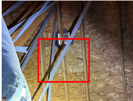
Area of prior repair viewed from attic
