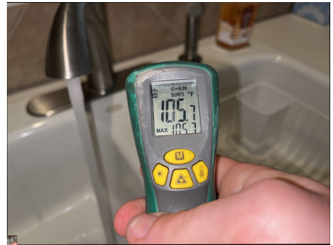
Hot water temperature
