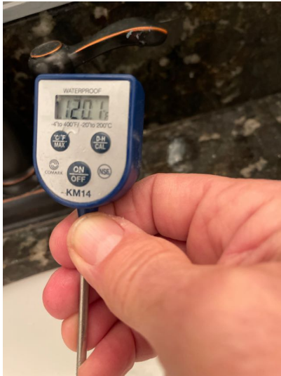
Plumbing System Water Heating Equipment
