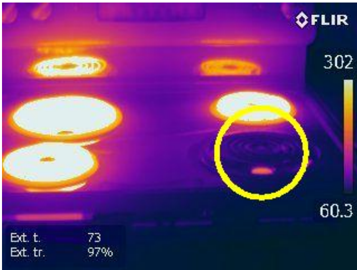
Right front burner was not functioning.
