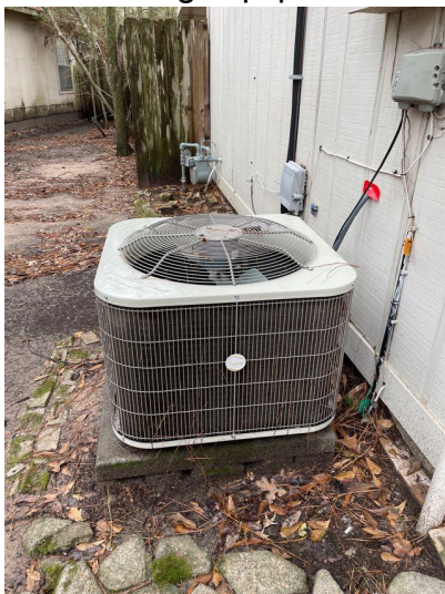
Heating, Ventilation and Air Conditioning Systems Cooling Equipment The Condensing unit manufactured by Payne in 2018. Unit appeared to be 3 ton, 14 SEER, using 410a refrigerant. Per the manufacturer's label, max amps on breaker should be 30. Per the labeling on the electrical panel, AC was connected to a 40 amp breaker.
