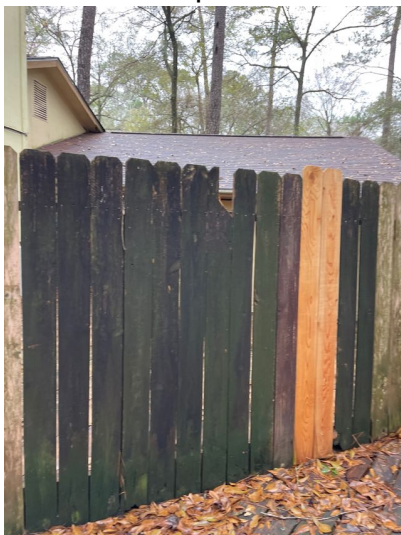
Fence in the back yard appeared to be weathered with damaged and rotted pickets, loose posts and loose panels.
