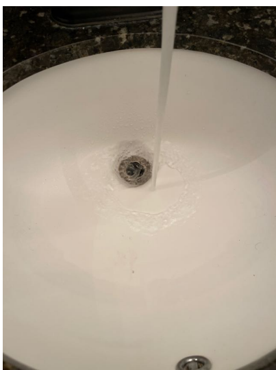
Sink stopper was not present in the upper bathroom.
