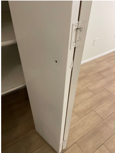
The pantry door and the upper bedroom closet bi-fold doors were missing a door handle.
