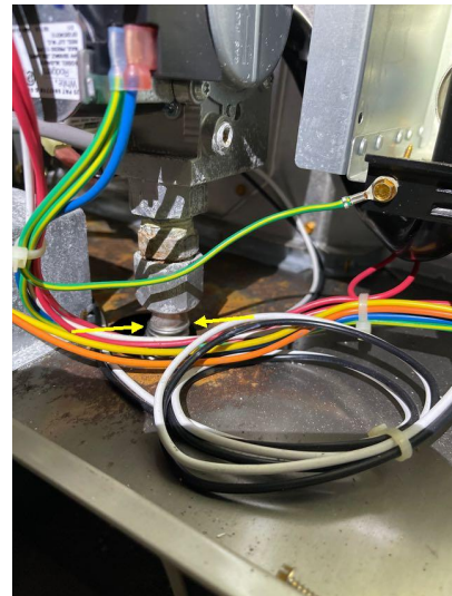
Flex gas line was entering the furnace and is not rated for this application. This connection should be hard piped.
