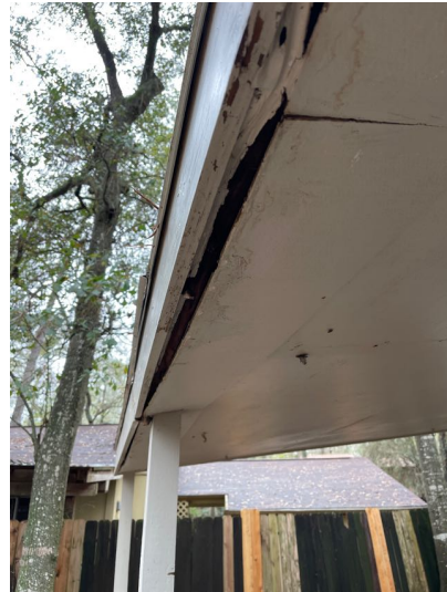
Fascia and soffit was rotted on the back deck cover. These areas are likely leaking from the roofing material on the deck cover.
