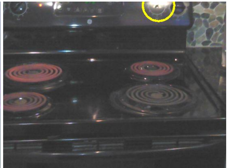
Temperature control knob was missing.
