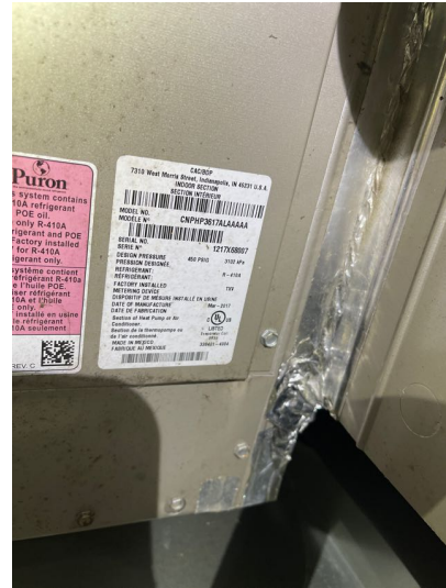
Heating, Ventilation and Air Conditioning Systems Cooling Equipment Evaporator unit manufactured by Carrier in 2017. Unit appeared to be 3 ton.
