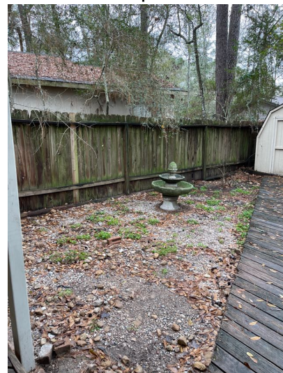
Fence in the back yard appeared to be weathered with damaged and rotted pickets, loose posts and loose panels.
