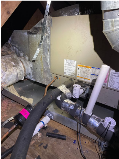
Heating, Ventilation and Air Conditioning Systems Cooling Equipment Evaporator unit manufactured by Carrier in 2017. Unit appeared to be 3 ton.
