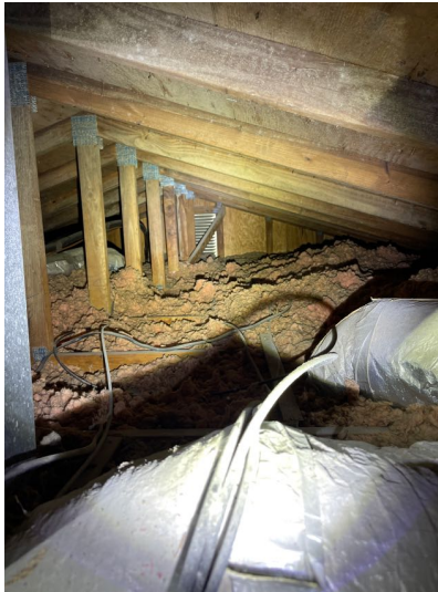
Structural Systems Roof Structure and Attic
