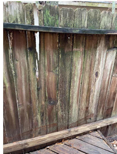
Fence in the back yard appeared to be weathered with damaged and rotted pickets, loose posts and loose panels.
