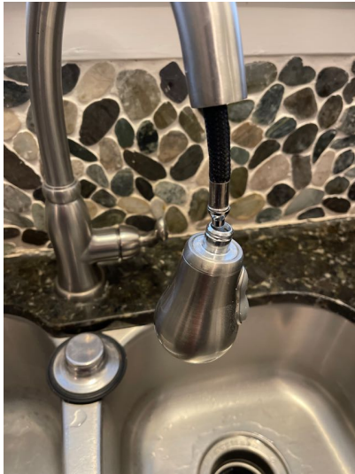
The kitchen sink fixture vegetable sprayer would not return to the stem.
