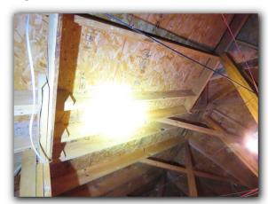
☑ Evidence of moisture penetration\*\*(Deficiency)\*\*(above the master closet); in need of repair by a roofing expert)
