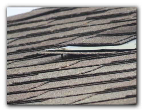
THERE IS VENTS AND FLUES WITH RAISED FLASHING THAT NEEDS TO BE PROPERLY SEALED DOWN BY A ROOFING EXPERT. \*\*(Deficiency)\*\*
