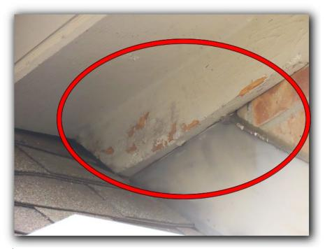
☑ Flashing is lifting, ill configured, or missing; and active roof leaks with water stains/patchwork on the master closet below. In need of repairs by a roofing expert. \*\*(**Deficiency**)\*\*
