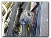
☑ DEFICIENCY- NO GREEN BOND SCREW PRESENT AS IS NOW REQUIRED; RECOMMEND EVALUATION AND REPAIRS BY A LICENSED ELECTRICIAN.\*\*(Deficiency)\*\*
