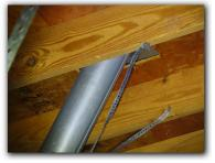
• THERE IS SOME RAFTERS WITH SEPARATION FROM THE RIDGE BEAM THAT IS ALSO COMMON WITH STRUCTURAL SETTLEMENT AND IN NEED OF EVALUATION AND REPAIRS BY A FRAMING EXPERT.\*\*(Deficiency)\*\*
