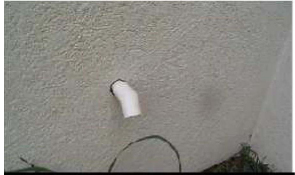
Fig. 1 Unsealed penetration
