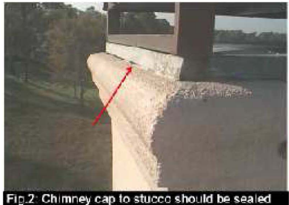
Fig.2: Chimney cap to stucco should be sealed
