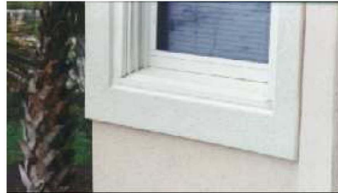
Figure 1: Typical inset window detail (sealed)
