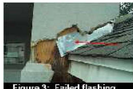
Figure 3: Failed flashing
