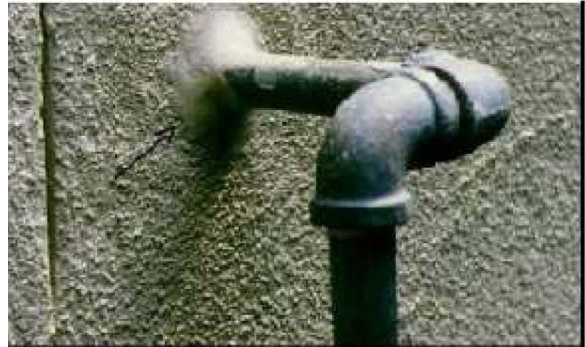
Fig. 2 Sealed pipe penetration
