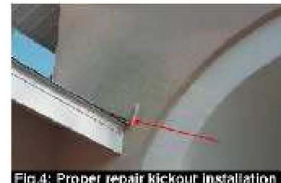
Fig 4: Proper repair kickout installation
