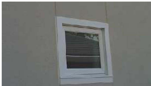
Figure 2: Typical outset window detail (sealed)
