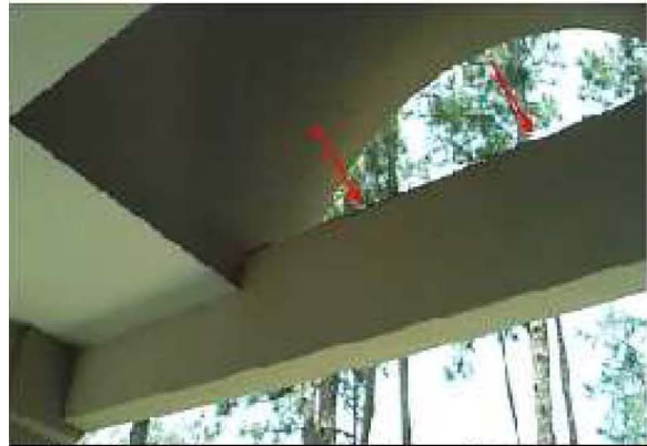
Fig. 2: Flat surfaces on top of beams
