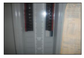
The breaker is oversized per data plate on side of A/C unit; 1st floor unit.
