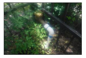
Water supply piping observed to be a mix of copper and plastic.
