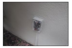
Improperly wired, 3 prong outlet not grounded or polarity reversed, including but not limited to; second floor master bath east side
