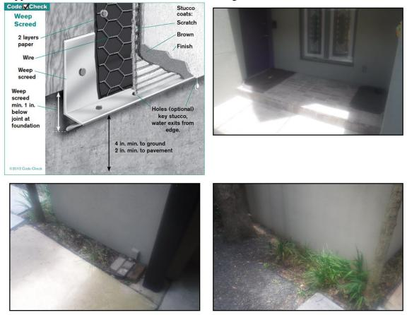
Bushes/trees/foliage should not contact the stucco siding of the house which can and will damage the protective stucco finish.
