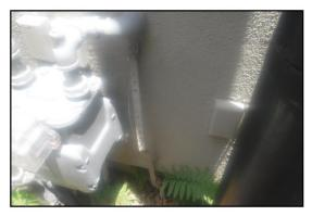
Exposed exterior gas piping not protected from corrosion as required per IRC 2603.3
