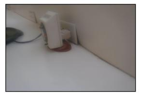
Recommend sealing all holes in interior walls to reduce air and water infiltration; kitchen counter, master bath.
