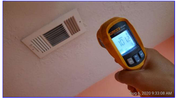
A. Item 3(Picture) Front left corner bedroom
