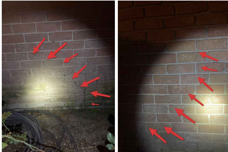
Exterior wall across from kitchen
