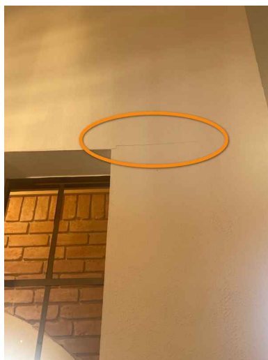
Foyer above front door
