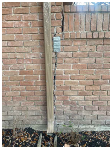
Exterior wall of Arbor, attached to master bedroom
