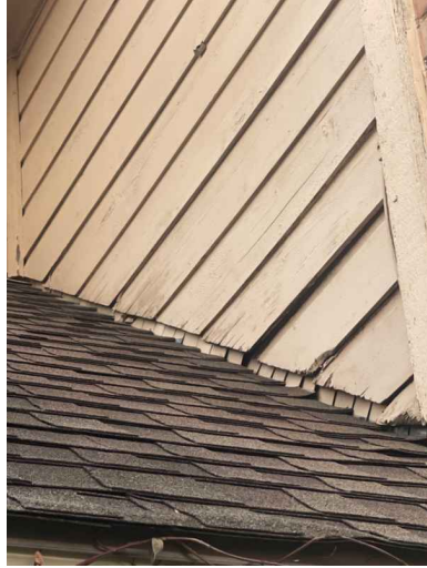
Roof wall intersection above downstairs office
