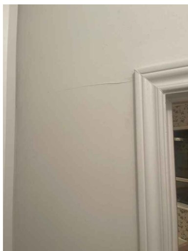
Master closet, right of master bathroom entrance
