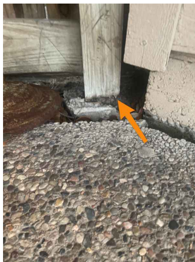
Fence between main house and garage
