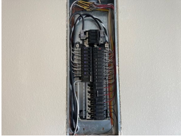
Main Panel: 200 amp, Located in garage
