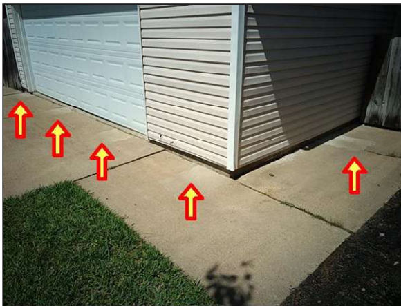
concrete patches from foundation work
