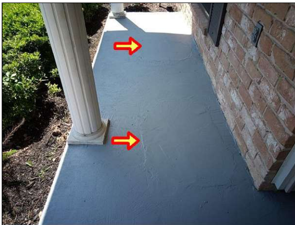
concrete patches from foundation work
