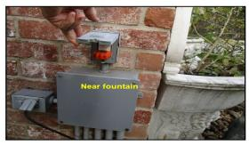
Multiple outlets are not secured well in the wall.
