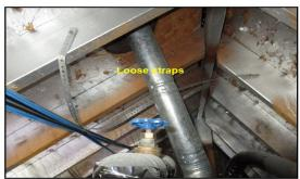
Improperly vented - vent pipe not properly aligned / secured at the top of water heater.
