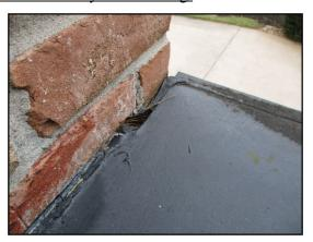
Observed rusted flashing; Above portica shea, and chimney cap rain deflectors
