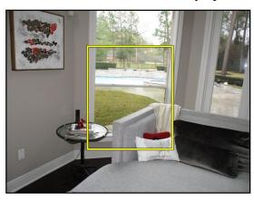
Window jamb alarm sensors need to be sealed with silicone seal to prevent water entry.
