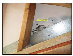
Hole and/or damaged roof decking observed in the attic, recommend repair to prevent damage/injury from a person walking on the roof; Near South dormer.
