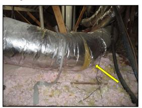
Observed unrated/labeled silver tape used on the HVAC duct system. This material does not adhere properly/well to the surface and allows excessive air loss. Recommend covering existing unlabeled silver-tape entirely with fiber-reinforced duct sealant such as "airlock" brand.
