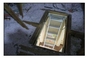
Inadequate attic walkway and/or platform to mechanical equipment in the attic. Code violation, [IRC M1305.1.3] requires 30-inch head clearance and a minimum 24 inch wide SOLID (no gaps or obstructions), floor to equipment for servicing and a 30 inch deep solid platform in front of the equipment.
