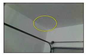
Observed cracks, repairs and/or repaired cracks in sheetrock observed in ceiling at one or more areas of house, possibly due to house settlement; second floor.
