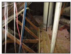
Water heater above master is difficult and could potentially be hazardous to access, recommend the addition of a railing to prevent a possible fall hazard.
