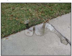
One or more spray heads are clogged and / or grass has grown over head, blocking / preventing proper operation.
