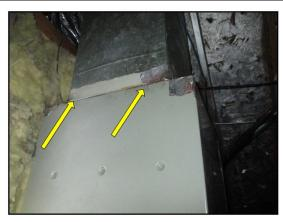
Observed multiple areas of damaged/ loose outer vapor seal on the flex duct in the attic.
