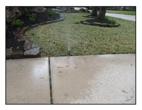
One or more spray heads need adjustment for proper yard cover and reduced over-spray on the house, fence, and paved areas.
