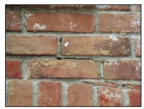
Cracks in brick / stone veneer and/or repairs, one or more locations, Recommend buyer take photographs of cracks, their location, and width [ruler across the crack] with a high-resolution camera that has a date stamp for future reference.
