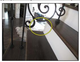
Space between railings does not comply with current industry standard, Per IRC 312.2, UBC 421.1.1, Requires spacing between intermediate rails do not allow passage of an object four inches in diameter. Recommend covering large openings in stair rails with temporary type nylon netting if small children are present in the house to prevent injury.
