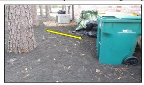
Soil level too high, in contact with siding and/or at/above brick weep holes at one or more locations around the house/garage. Promotes wood rot and is considered a conducive condition to termite activity.
