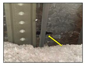
Radiant barrier paint is peeling/falling at multiple locations.
