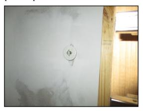
Gas valve improperly located more than 3 feet from unit, difficult to access, and/or on the opposite side of the unit; master bedroom.
