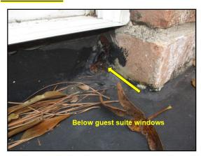
Observed masonry counter flashing missing or improperly installed Above portica shea.
