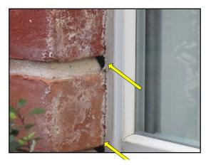
Need sealing/caulking around all holes and exterior siding penetrations on top and both sides, (*leave the bottom open*) to prevent water entry. Including but not limited to dryer, bath and range top vents, light fixtures, etc.
