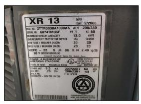
Note: Unit using older refrigerant (R22). This refrigerant is no longer being manufactured and will become very expensive in the near future.
