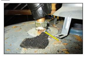
Gas and hot/cold water lines are not properly bonded near the water heater. This does not comply with the most recent electrical code.
