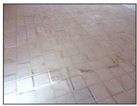
Grout/caulking needed at vertical tile corners, cracks in tile and/or mortar between tiles, to prevent water entry behind the wall; Pet bath/ shower
