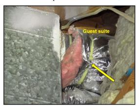
Observed filters in return air vent(s) AND at HVAC in attic. It is recommended to install air filters EITHER in return air chases OR at HVAC in attic. Installing filters at both locations can restrict air flow cause high head pressures at HVAC unit in attic.
