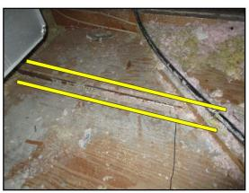
Recommend insulation of exposed water lines in the attic.
