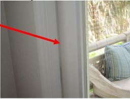
Top latch to French door is not properly align and or is stuck and does not function.
