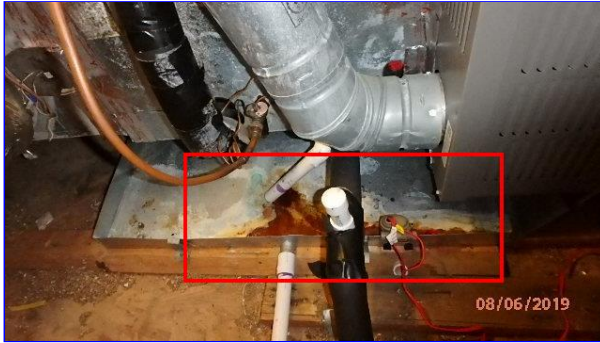
Water was detected in the safety pan of the DOWN STAIRS AC unit
