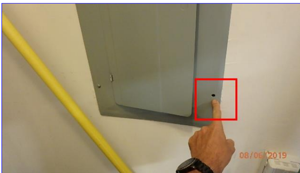
missing fastener
