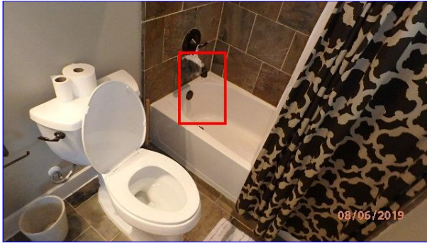
Shower diverting valve did not operate properly.
