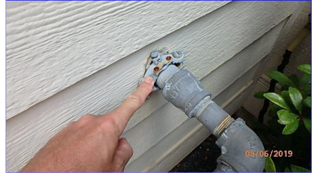
The bonding conductor should run to the grounding connection at the service equipment, this could not be verified during today's inspection.
