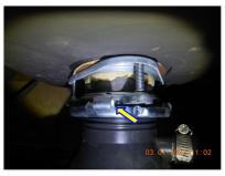
$\square$  The food waste disposal connection clamp is not locked into place at the sink flange. Disposal vibration may cause the unit to leak or detach at the sink connection.
