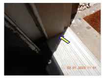
☑ Caulking around the door missing or deteriorated was noted. Some Examples: Front door.
