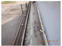
☑ Window drainage ports obstructed with dirt and debris. Window drainage ports and other components should be cleaned on a annual basis. Otherwise, drainage ports can be blocked allowing water to back up into the wall area below the windows.
