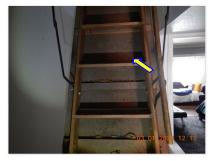
☑ Disappearing attic access ladder ceiling panel is not insulated at the attic.
