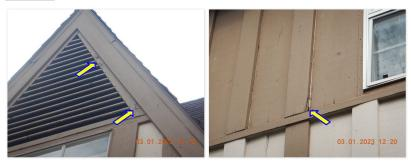
☑ Cement board siding and/or trim damaged/deteriorated.
