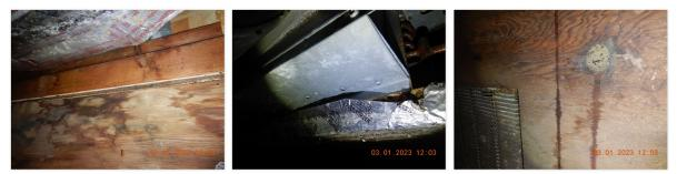
☑ Signs of moisture at the A/C equipment and access panel were noted at the time of inspection. DRAIN LINES:
