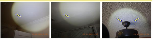
Cracks/damage/repairs in the ceiling drywall observed.
