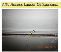
☑ Disappearing attic access ladder is not sealing properly at the attic.
