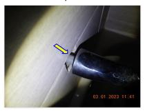
☑ A gap between the wall and tub fixture was noted at the 2nd floor bathroom.
