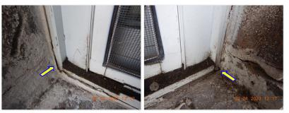
Caulking around exterior windows deteriorating.
