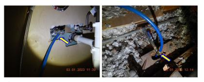
$\square$  Special notice: we observed some original galvanized pipe has been replaced, therefore the process of replacing the galvanized pipe has started. We encourage any potential home buyer to take into consideration the cost associated with replacing the galvanized pipe before any final purchase decisions are made.
