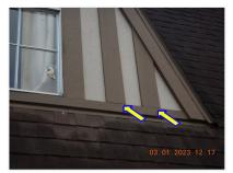
☑ Caulking is needed at all joints and unsealed seams in the siding. CAULKING:
