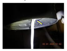
$\square$  The food waste disposal whip cord is not properly secured at the clamp at the base of the food waste disposal.
