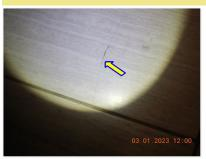
☑ Broken or cracked floor tiles observed at some locations.
