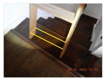
☑ Disappearing attic access ladder is missing the bottom step.
