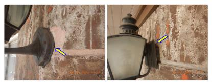
☑ Caulking/sealant is missing around the exterior light fixtures.
