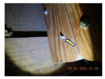
☑ Disappearing attic access ladder bolts are missing nuts.
