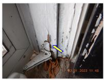
☑ Door and/or door jam casing deteriorated from weathering was noted. Some Examples: Back patio.
