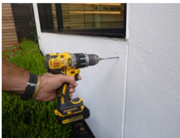
Drill two small (3/16 - 1/4") probe points for moisture probe access
