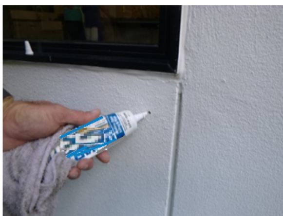
Seal holes with approved exterior caulk
