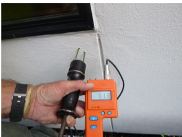
Take moisture reading with meter
