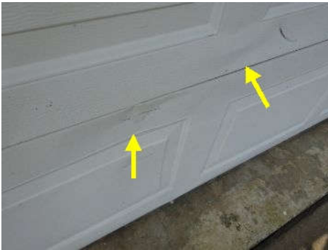
Doors have dents in several locations.
