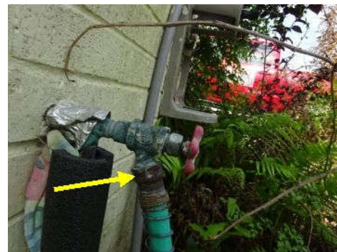
There are no back flow prevention devices installed on the exterior hose bibs, does not meet "current industry standards".
