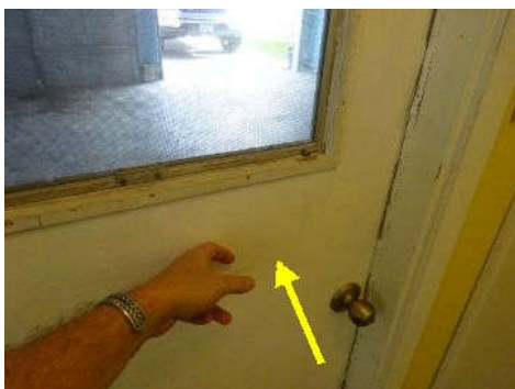
Door between garage and home is not a fire rated safety door. does not meet current industry standards.
