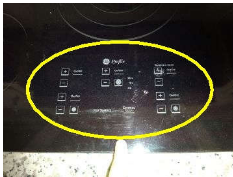
Cook top did not respond to controls.
