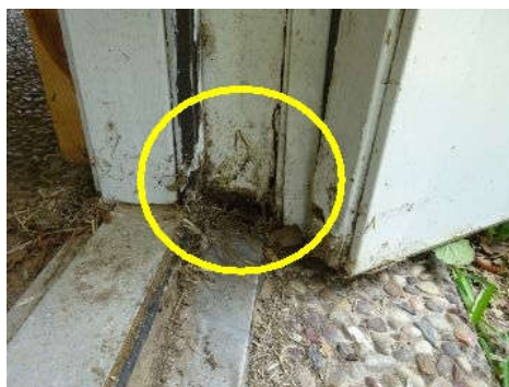
Observed wood rot to lower area of door frame at rear exterior entrance door to porch.
