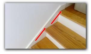
Damaged/Raised flooring was noted in living room hallway from possible moisture penetration . Recommend evaluation for repair
