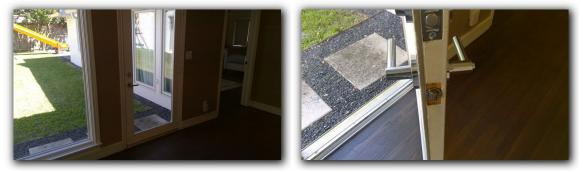
The middle rear exterior door shows signs of moisture penetration and elevated moisture meter readings (99.9%). Recommend evaluation for repair of all associated components by a qualified tradesman
