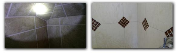
Hairline cracks were found on the interior of the property as evident of settlement. The cracks can be repaired if desired for cosmetic purposes.
