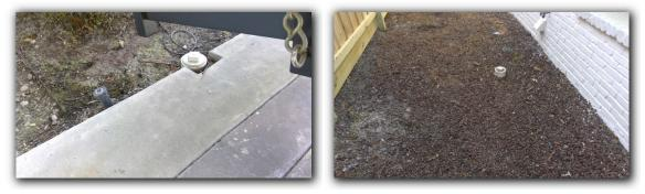
Building Codes, TREC Standards, Installation Standards or Safety Issues ☑ PVC piping exposed on exterior not painted to protect from UV rays ☑ Improper style drain material installed at fixture, i.e. missing smooth rigid pipe.
