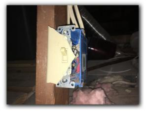
Aluminum neutral conductor was found at the neutral bar and i could not determine the what it went to. Recommend evaluation by a licensed electrician
