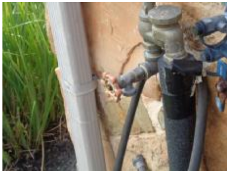
Backflow missing
