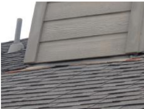
Rusted flashing
