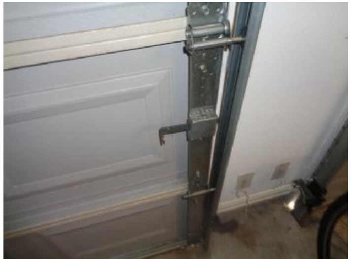
Manual lock not disabled with the presence of a garage door opener
