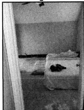
Living room into master bedroom
