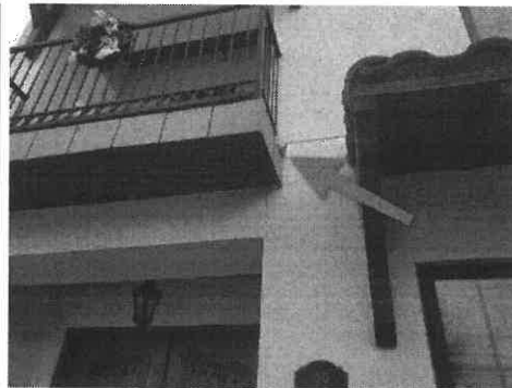
Corner flashing
