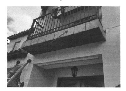
Note: EVERY balcony on this home is improperly flashed. Your inspector has failed to identify the missing drip edge flashing on each balcony. The drip edge is needed to allow water to divert from the face of the balcony.
