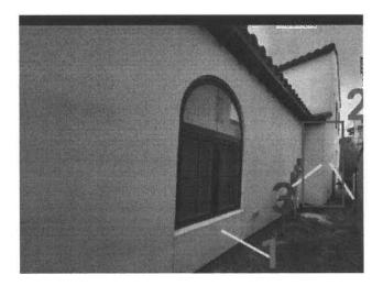
Note: Your inspector has failed to indicate if there is missing or improper kick out diverter flashings at the stucco to roof intersection above probe location 2. We will inspect those on our own and if they have failed or are missing, a cost range to replace them will be \$0 to \$500.00 in addition to the proposal amount.
