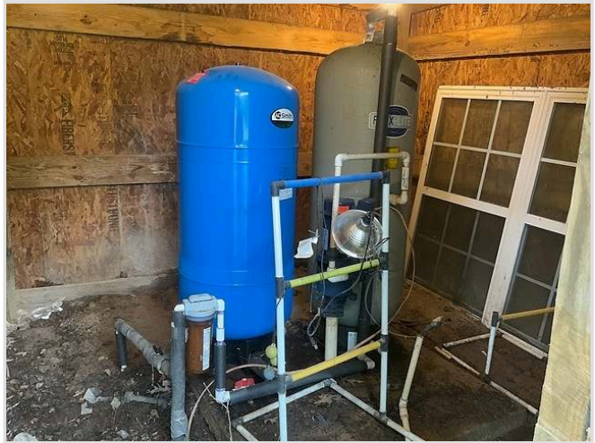
Metal/fiberglass tanks
