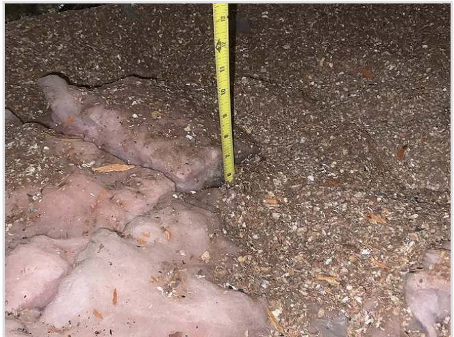
Insulation depth (approximately 12" - 14")
