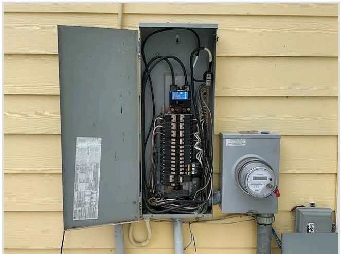
Panel cover removed for inspection
