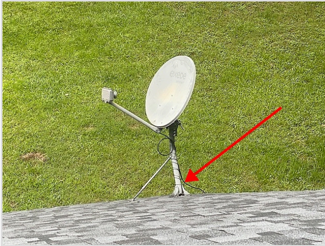
Installed over shingles
