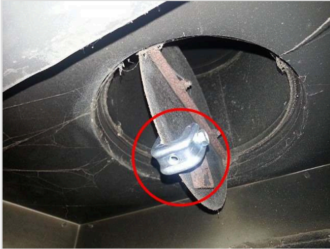
Damper clamp example
