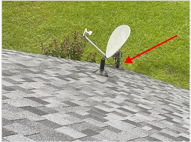
Installed over shingles
