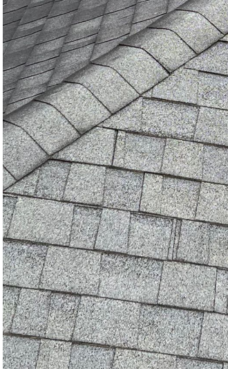
Picture of roof
