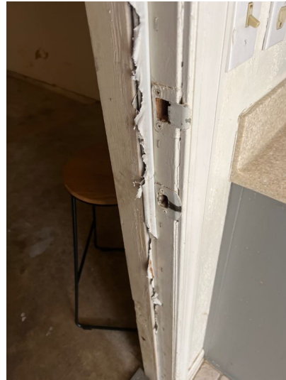
Garage door noted with Damaged weatherstripping
