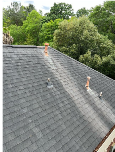
Picture of roof
