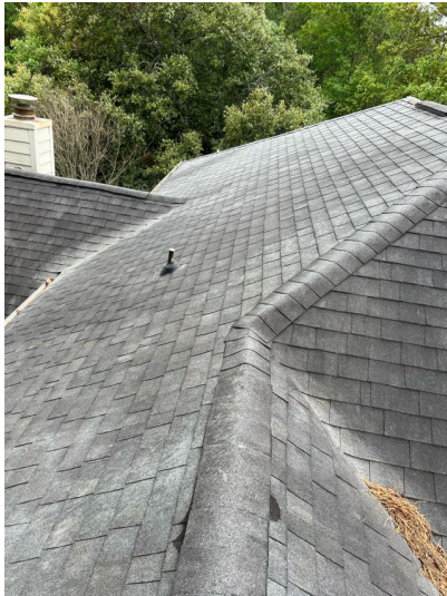
Picture of roof
