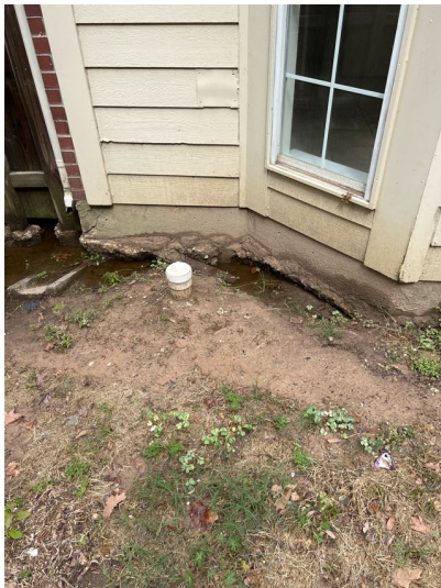
Low soil observed at one or more sides of the structure and recommend additional backfill.
