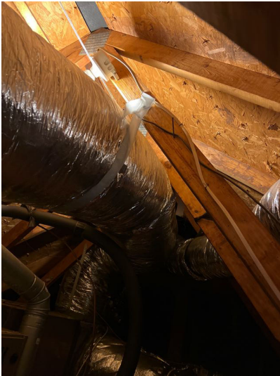
Picture of attic space
