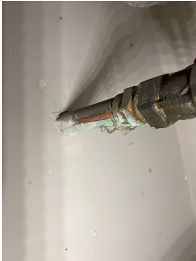
One or more of the exterior hose bibs {faucets} was observed to be leaking
