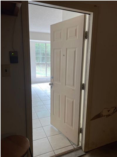
The garage entry door was not equipped with a self closing device.
