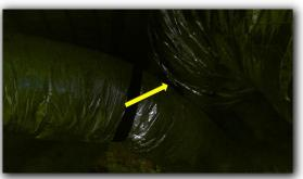
A/C duct work should be strapped up off of floor with 1  $\frac{1}{2}$  " straps at no more than 4' intervals,  $\frac{1}{2}$  " or less sag, per foot, between straps and three straps per turn without crimping and restricting duct work around or over framing.
