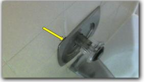
Caulk, grout caulk, or grout, as needed, all cracks at all bathroom shower wall/ tub surround corners, at tub, at ceiling, curbs, steps, and between tiles to prevent moisture
