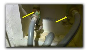
Non-sealed escutcheons at shower walls at all bathrooms should be caulk/sealed to prevent moisture penetration. Such as shower arm escutcheons, tub spouts, faucet controls..etc.
