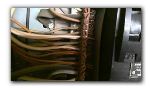
No conduit connector bond from meter to panel box noted, which was not required when home was built.
