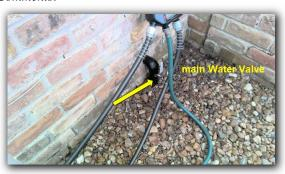
Recommend insulating all galvanized water supply lines where exposed in attic or exterior of house and periodically recheck for possible leaks and reduced water pressure due to build up of deposits in lines. The supply lines appear functional and stable with no obvious excessive deposits or leaks at this time, where accessible and visible.
