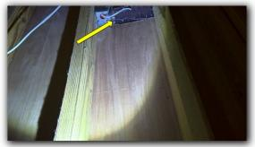
Vent in full bathroom upstairs appears to have very minimal flow. Recommend having a licensed hvac technician evaluate and repair or replace as needed.
