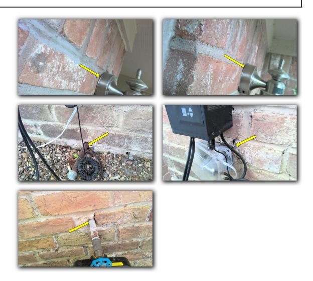
Seal and paint exterior siding/trim/soffit/fascia at nail heads, overlap edges, butt joints, separations, vertical joints.... etc. to prevent water penetration at dings, scuffs and holes to extend life.
