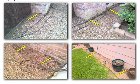
French drains noted at backyard/sides. Recommend buyer monitor these drains to ensure proper drainage during or after rainfall. Properly clean al drain basins and/or properly secure/replace loose or damaged grates, as needed.
