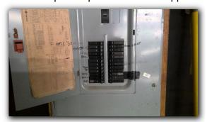
AFCI breakers are not noted at all living areas where required, per current electrical code, however these or not all were not required when home was built. AFCI breakers are not always tested by inspector when computers, alarm systems, other electronics....etc are on circuit or other circumstances.
