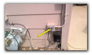
Recommend receptacle be installed at exterior/interior HVAC unit for servicing and repair, as is currently a building standard.
