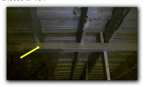
Collar ties should be installed at every other rafter set in upper 1/3rd of attic space, where noted as missing.
