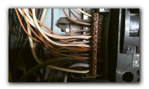
Move neutral double tapped wire to separate and single tapped lugs at neutral buss or ground buss bar as required in panel box.
