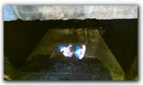
Bricks in back of firebox need pointing up with fire clay.
