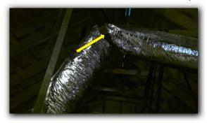
Install insulation or other approved material between ducts coming in contact with one another to prevent possible condensation forming as needed in attic.
