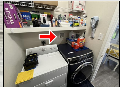
Main Water Shut Off
