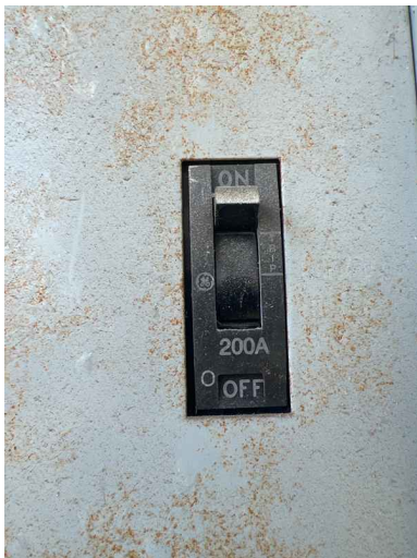
Main Service Panel Amperage: 200 Amp
