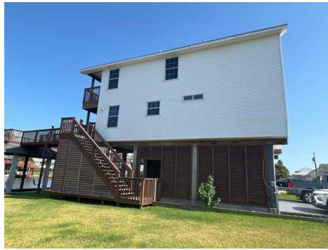
North Facing side
