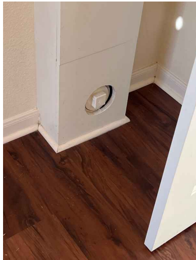
Location of Main Clean-out: Inside front entry
