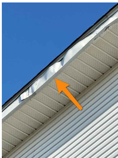
North Facing side
