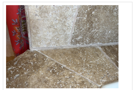
(5) Tub or shower requires caulking at the corners of shower walls and at the base of tiled shower.
