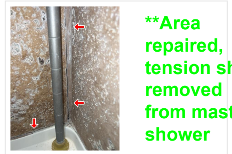
(5) Tub or shower requires caulking at the corners of shower walls and at the base of tiled shower.
