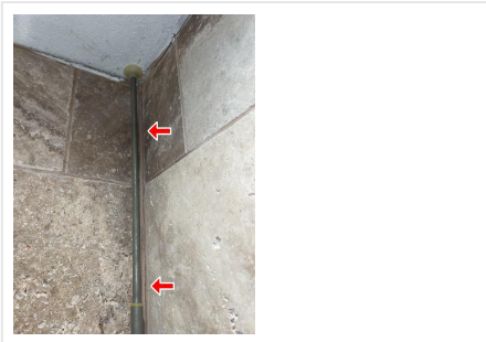
(5) Tub or shower requires caulking at the corners of shower walls and at the base of tiled shower.
