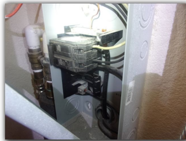
The panel in the laundry was in good condition.
