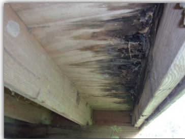
Previous moisture damage noted under the master tub
