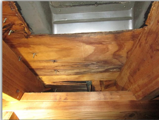
Evidence of prior water penetration in multiple locations.
