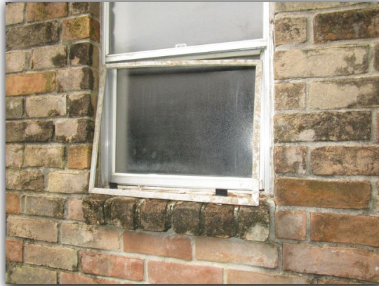
Multiple windows need re-caulking to brick.
