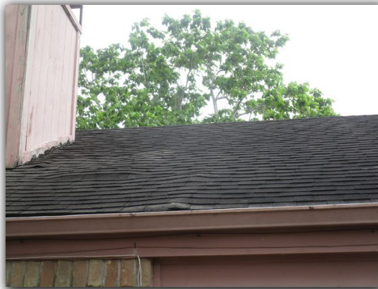
Drip edge and flashing's were loose, rusted and/or showed evidence of prior water penetration underneath the installation.
