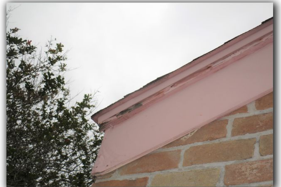
Drip edge and flashing's were loose, rusted and/or showed evidence of prior water penetration underneath the installation.
