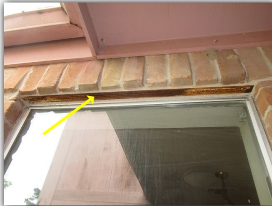
Some windows needed lintels repainted.
