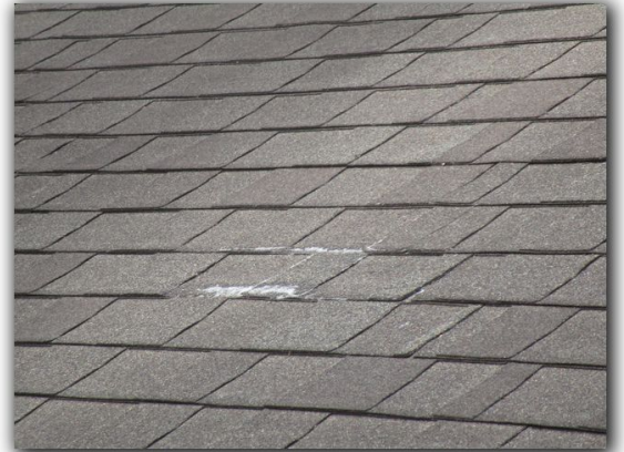
Uneven roof decking was observed in the rear of the house.
