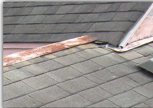
Drip edge and flashing's were loose, rusted and/or showed evidence of prior water penetration underneath the installation.
