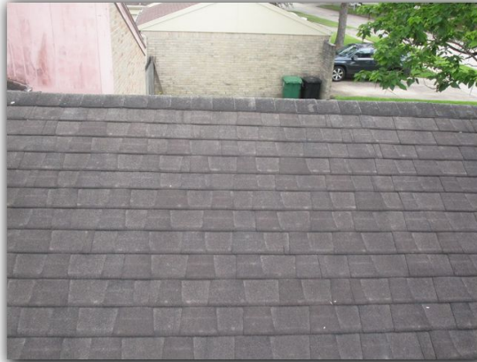
Uneven roof decking was observed in the rear of the house.
