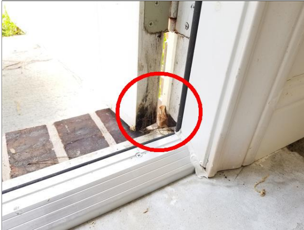
Wood rot/water damage forming on base of door
