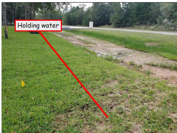
Front of home at road ditch
