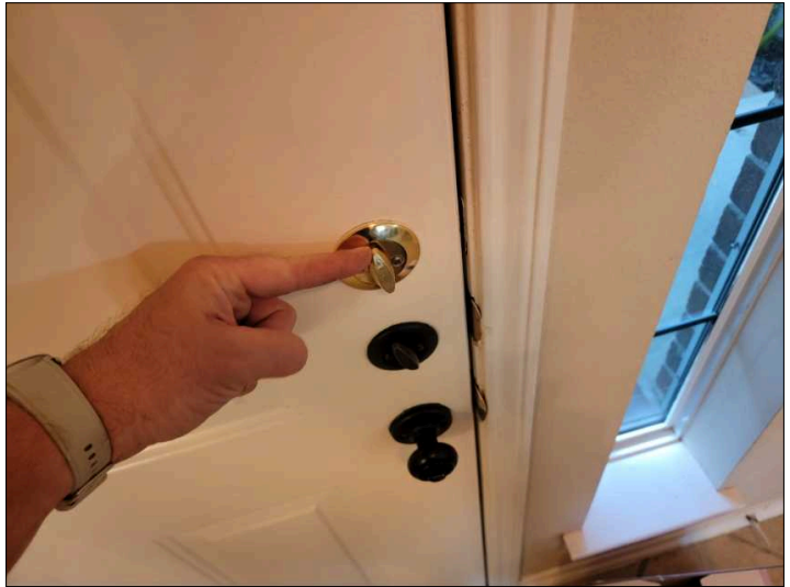
Deadbolt doesn't fully engage at garage door
