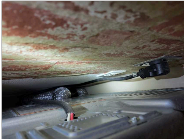
Could not fully inspect the dryer vent, due to access.
