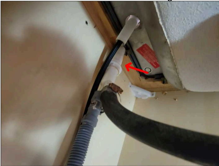
Air gap device is present under sink. Should be above counter so that it can be monitored for leaking.
