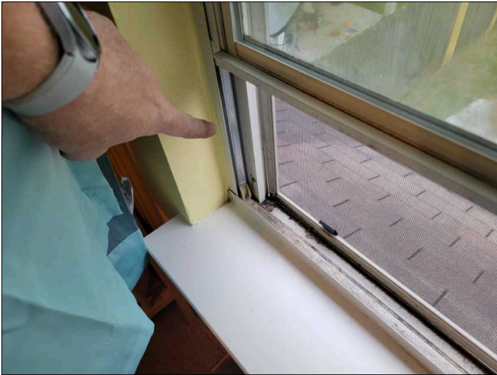
Broken or damaged balancers (springs, spirals, or friction rods) present. These hold the window up.
