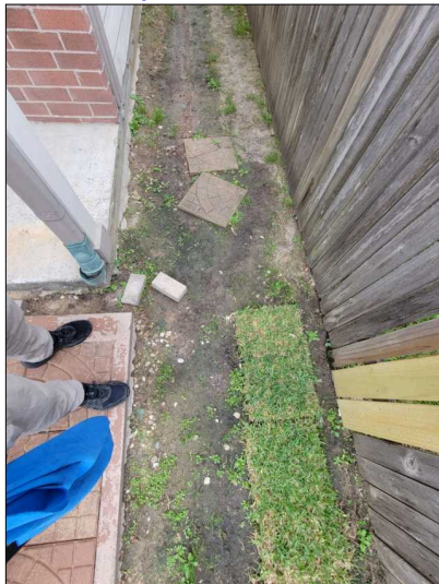
Ponding water noted in low areas of yard.
