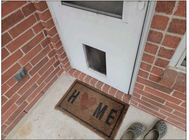
Pet door noted
