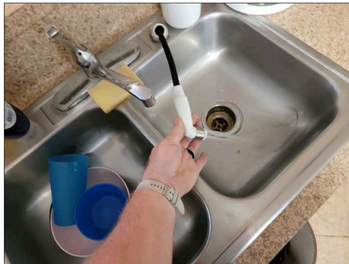
Poor water flow at vegetable sprayer.
