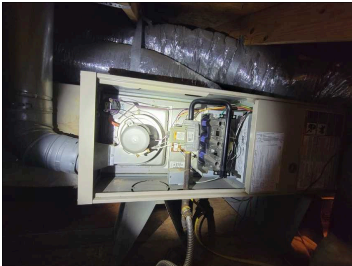
Furnace visually inspected and checked.
