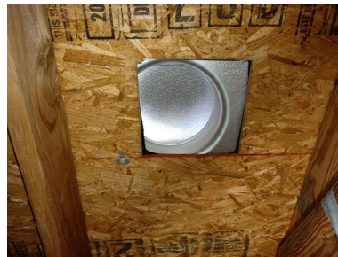
Roof Vent (from Attic)
