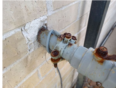
Gas Line Bonding
