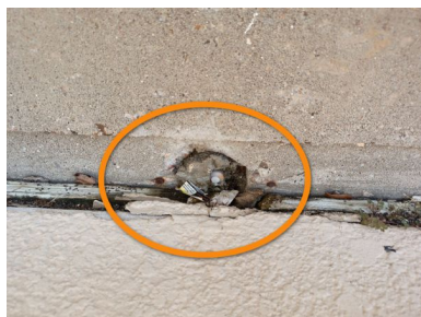
Garage Right Exterior
