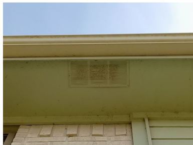
Soffit Vents
