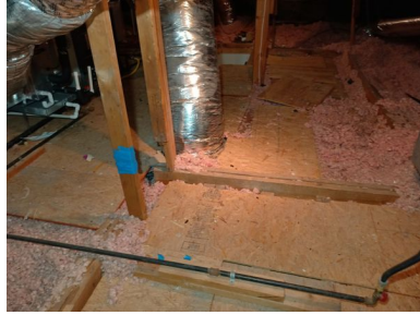
Approximate Average Depth of Insulation: More than 14 Inches
