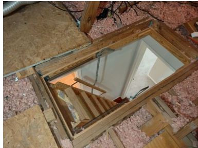
Type of Attic/Roof Ventillation: Roof and Soffit Vents
