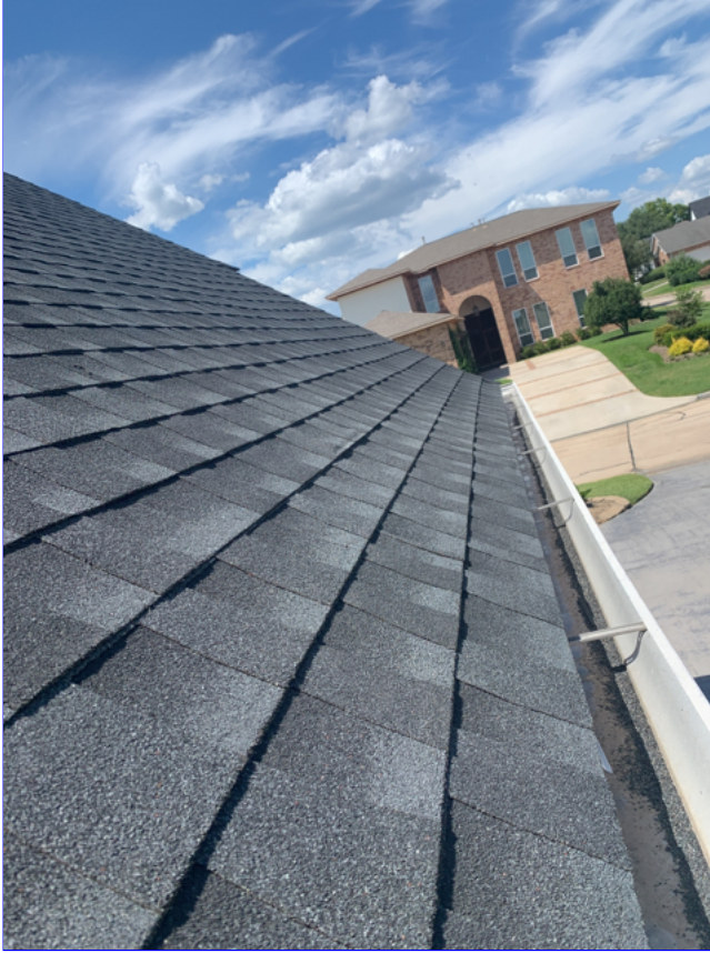
C. Item 3(Picture) The roof covering, is not new and shows signs of wear consistent with its age.
