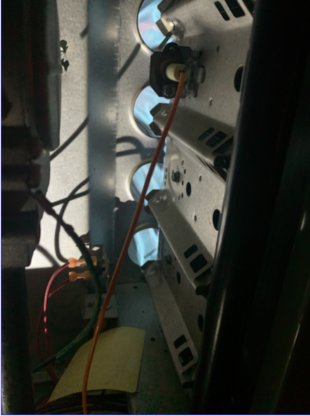
A. Item 1(Picture) Furnace burners
