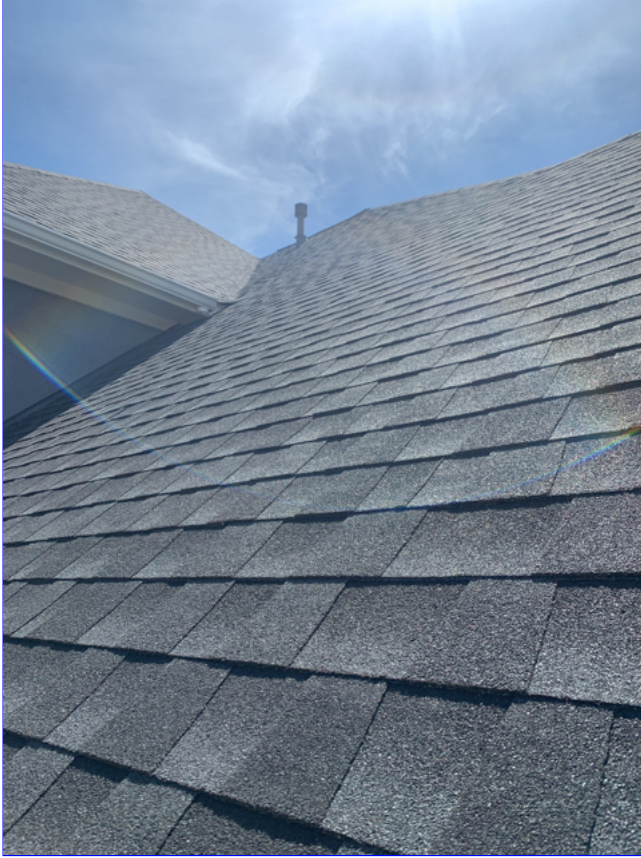
C. Item 2(Picture) The roof covering, is not new and shows signs of wear consistent with its age.
