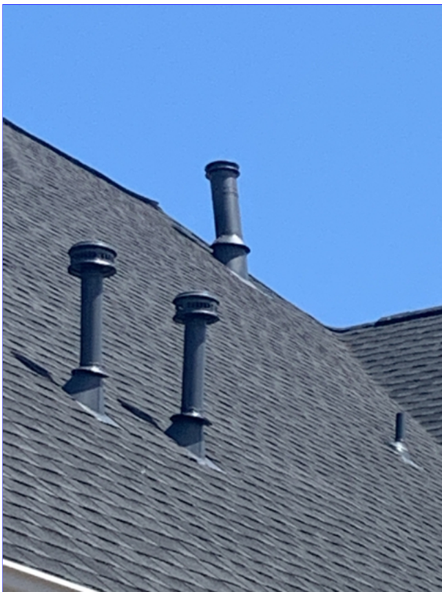
C. Item 4(Picture) The roof covering, is not new and shows signs of wear consistent with its age.
