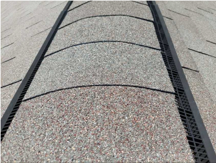
Picture of roof
