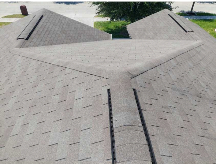
Picture of roof
