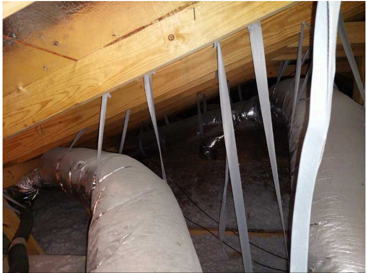
Picture of attic space
