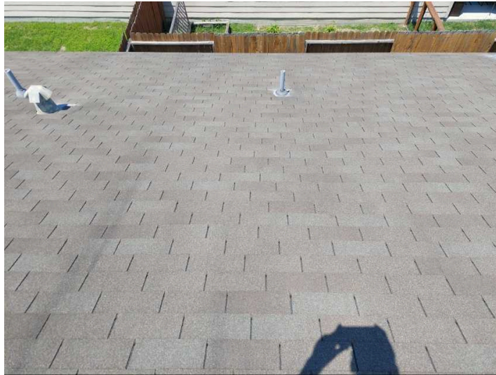
Picture of roof
