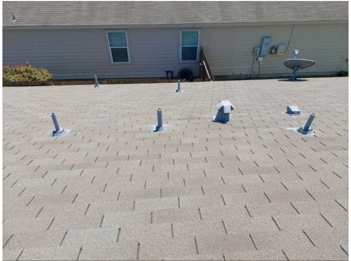
Picture of roof
