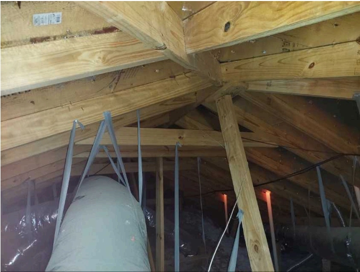
Picture of attic space
