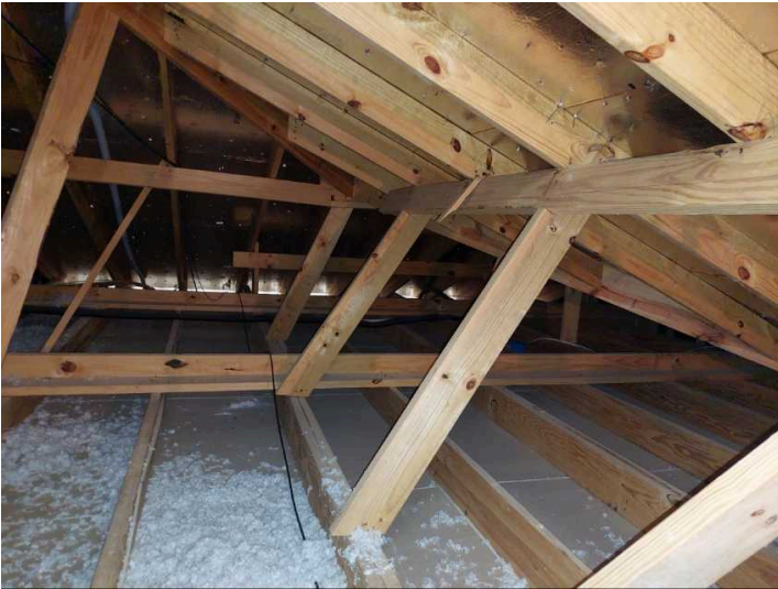
Picture of attic space
