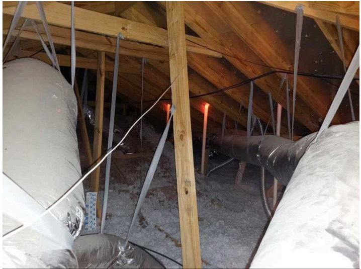
Picture of attic space
