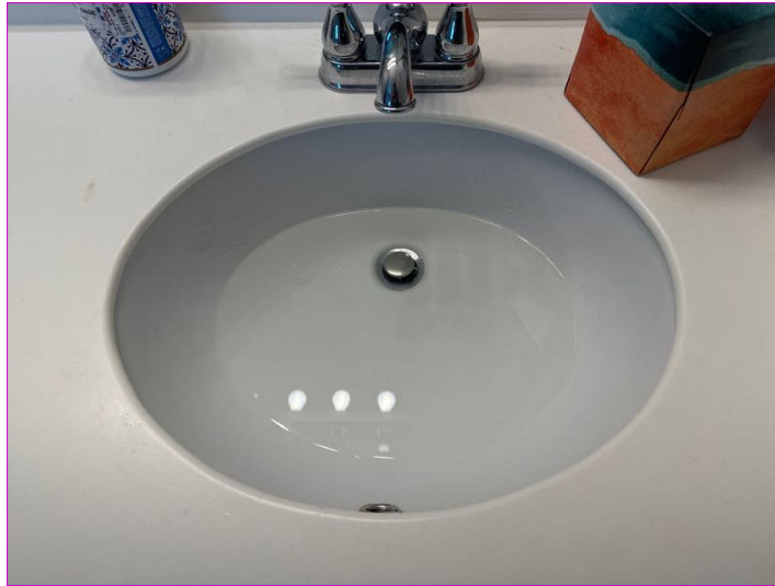
Slow sink drain (master bathroom)
