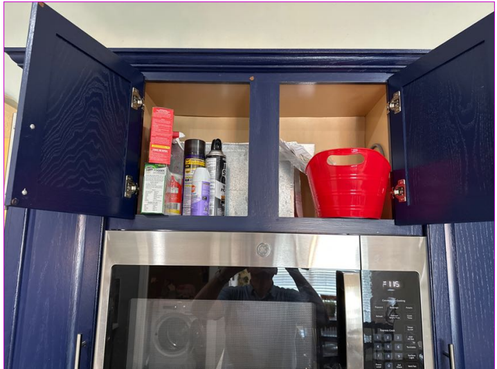
Outdoor exhaust duct OK
