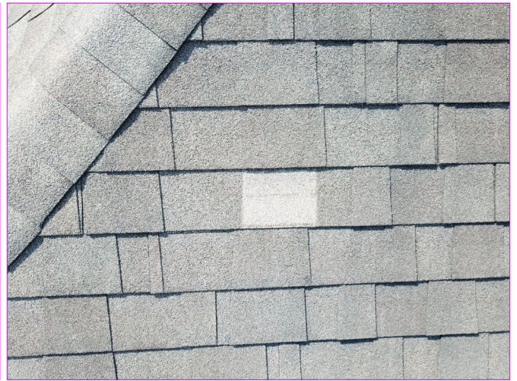
Damaged shingle
