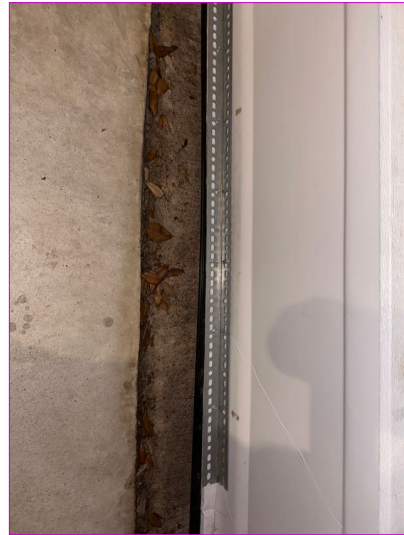
Repaired garage door
