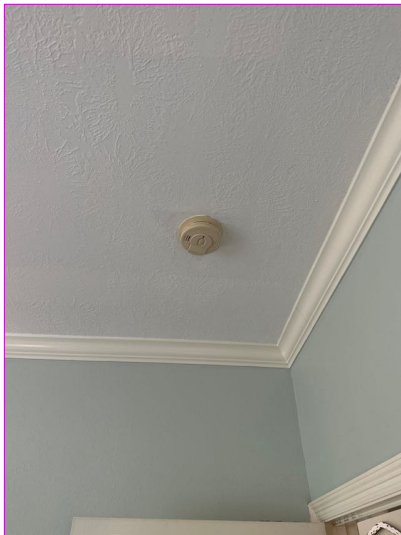
Replace old smoke detectors
