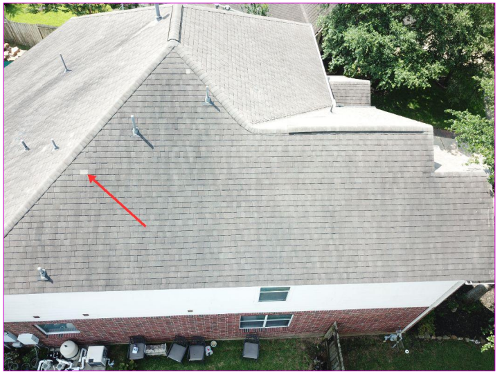
Damaged shingle
