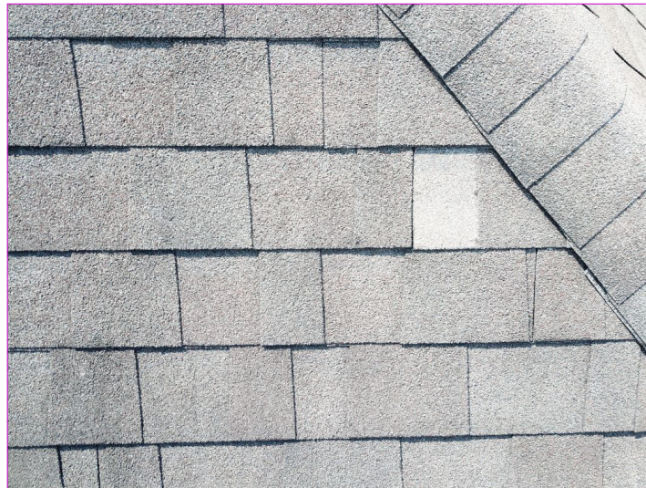
Damaged shingle
