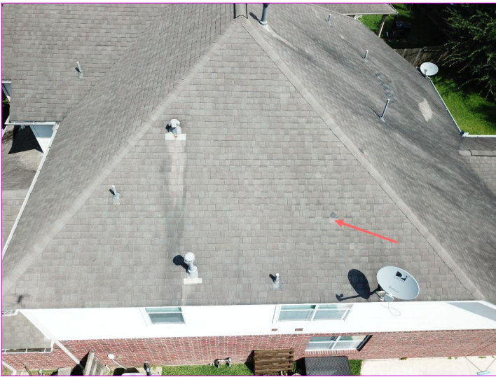
Damaged shingle
