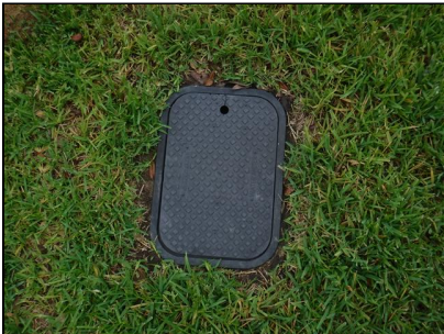
Water meter located right side of residence.
