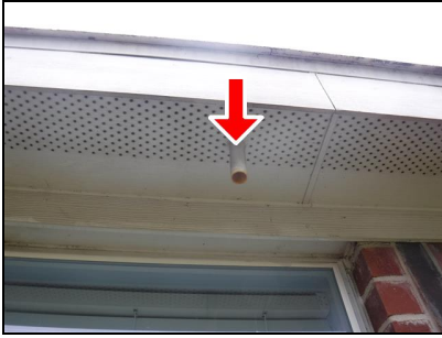
A/C secondary drain located right side of residence.
