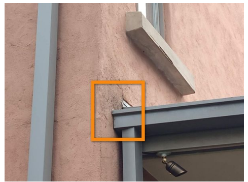
HS file photo illustrating kickout flashing
