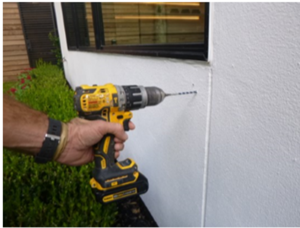
Drill two small (3/16 - 1/4") probe points for moisture probe access
