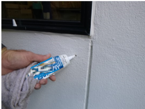
Seal holes with approved exterior caulk
