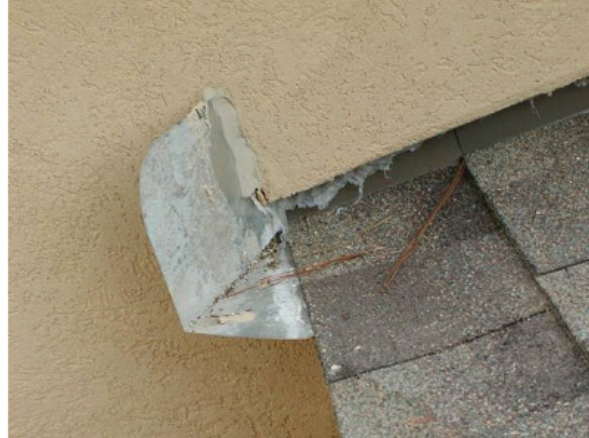
HS file photo illustrating kickout flashing
