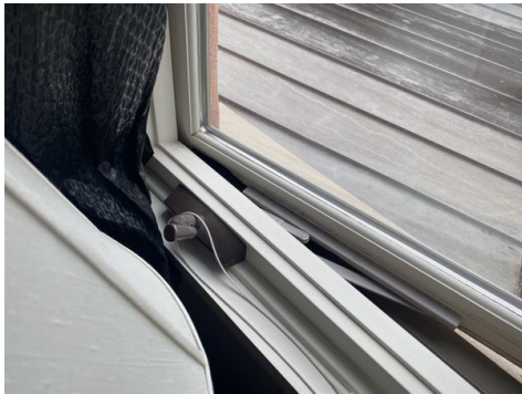
North West Bedroom Repaired
