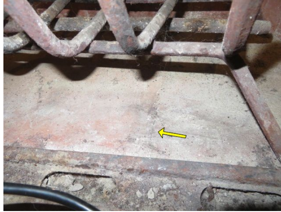
The rail for the fireplace screen is loose.
