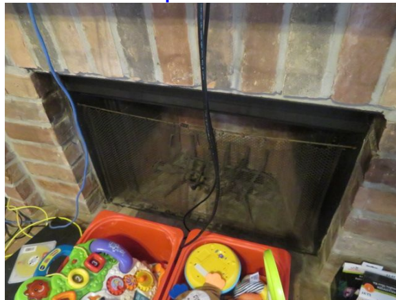
The rail for the fireplace screen is loose.
