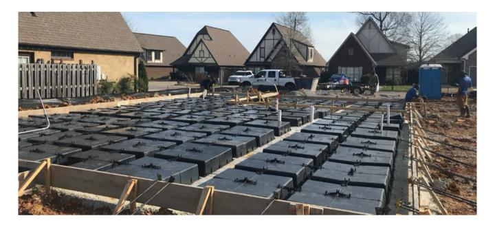
A Waffle Slab Foundation, also known as a ribbed slab foundation, is an above-ground concrete foundation that is designed to withhold incredible load-bearing capacity for single family, multi-family, and light commercial structures.
