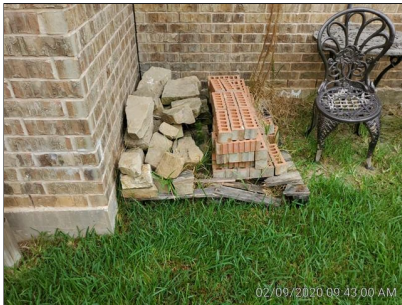
Wood to Ground Contact
