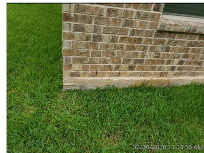
Rear: Corner Pop, non structural crack
