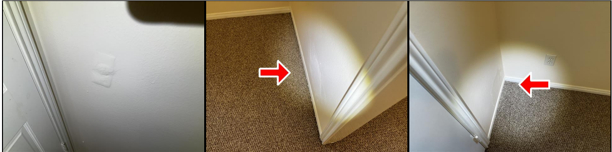
Noted areas of the walls that have prior repair.
