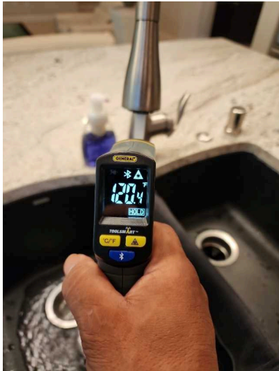
Water heater temperature
