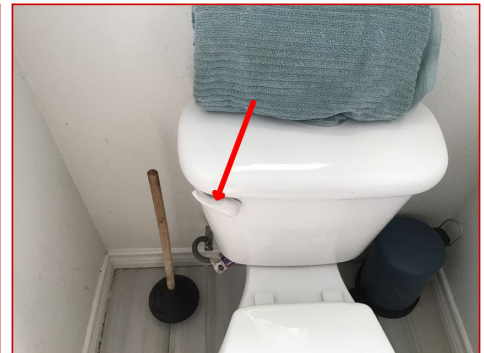
Sticking handle, attached bath
