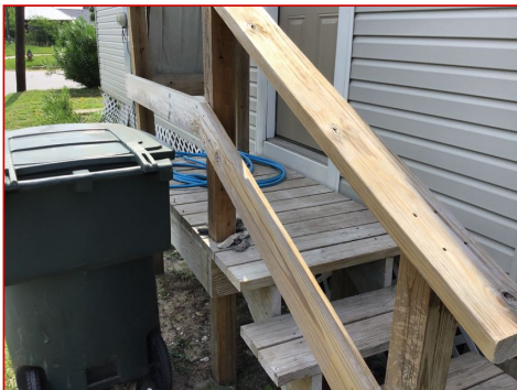
Climbable guardrail and handrail
