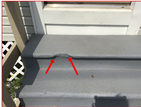
Damaged tread
