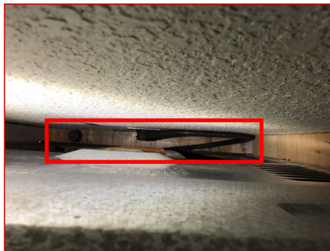
Missing anti tip bracket
