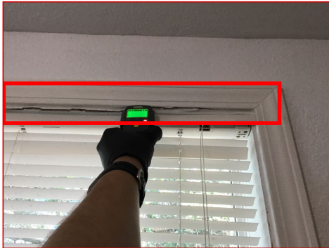
Evidence of moisture intrusion, rear bedroom
