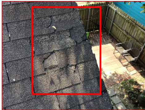
Damaged shingles
