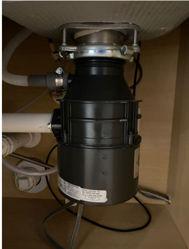
General Photos of Range Hood/Exhaust System(s):
