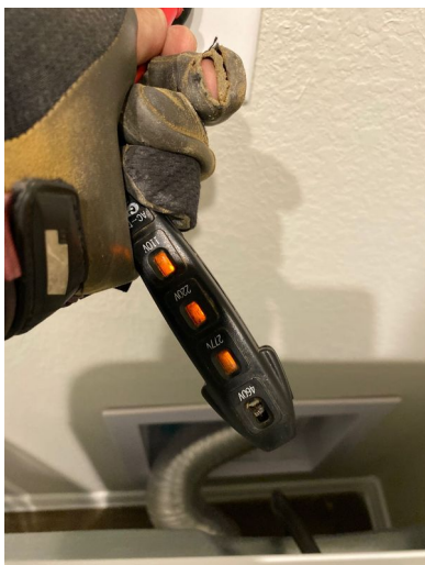
General Photos of Grounding Systems:
