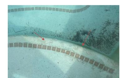
2. Expansion joint: Expansion joint/mastic joint/deck-o-seal is gone. This is an epoxy joint that prevents water from rain, overflow, etc, from getting inbetween the structure of the pool, and the deck. This prevents deck shifting and should be replaced every 5-8 years, as needed.
