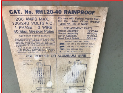
Federal Pacific Stab Lok panel, 200 amp max rating
