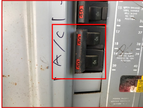
AC on 50 amp breaker, mfg label states max allowed of 40 amps
