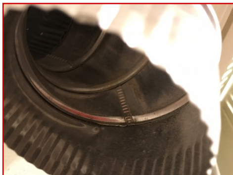
Dryer vent appears ok
