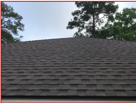
Laminated (architectural) shingles
