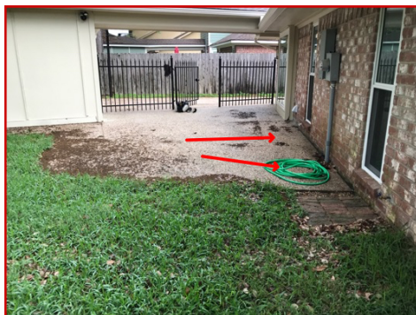
Rear patio appears to slope towards the house
