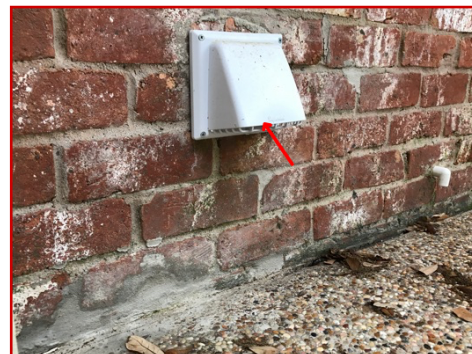
Dryer vent has a screen on it
