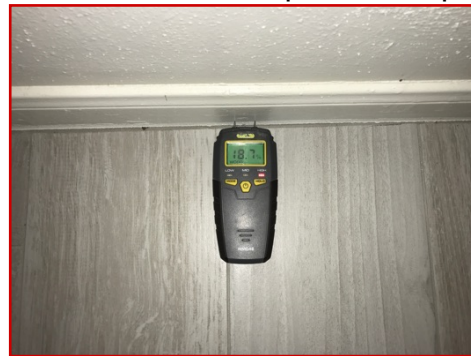
Elevated moisture levels in laundry room and kitchen
