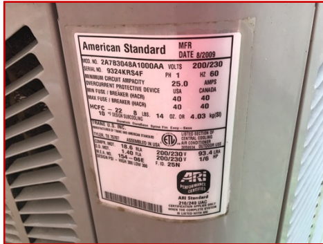
American standard 4 ton, R-22 coolant, max 40 amp breaker, mfg 2009
