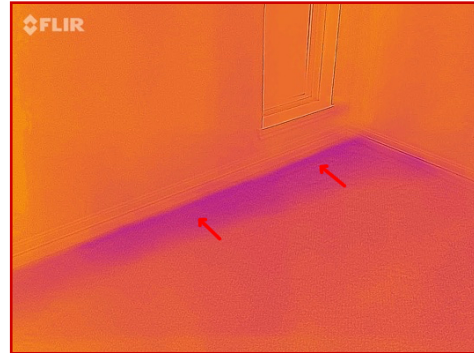
Carpet in master bedroom tested with elevated moisture levels
