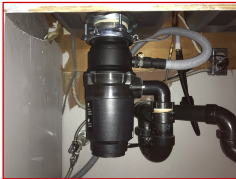
Disposal appears ok
