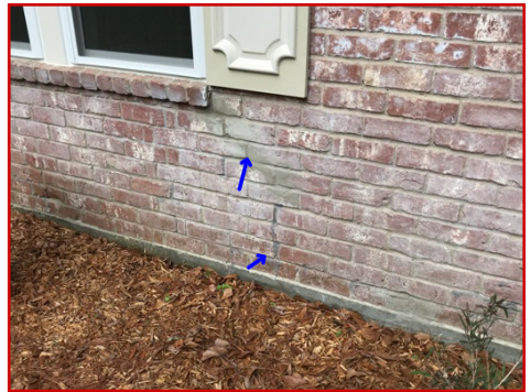
Multiple brick repairs
