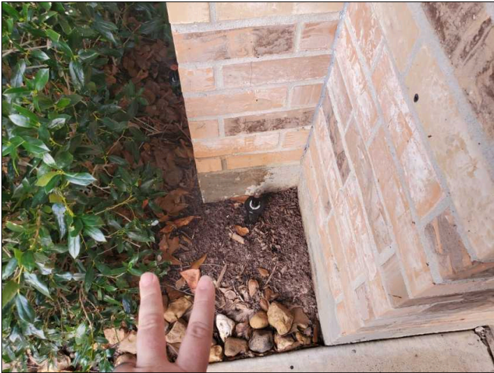
Zone 2 sprinkler spraying house, needs adjusting
