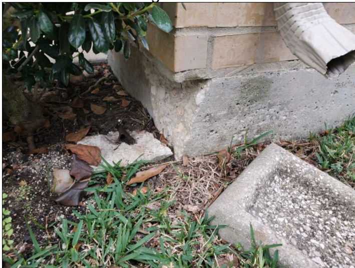
Corner pop noticed. Corner sections of the foundation are not supported as much as rest of foundation. This is not typically an issue, but take notice if cracks begin to form in bricks or mortar above corner pop.
