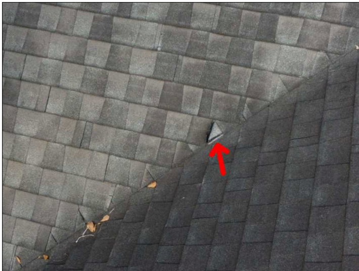
Shingles are missing / torn
