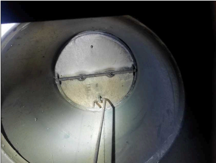
Damper missing its damper clamp. This clamp keeps the damper from being fully closed, in the event fireplace is lit, and CO2 has chance to enter into house.
