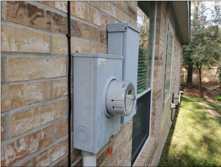
Panels that attach to exterior walls should be sealed on top and sides, but not bottom.
