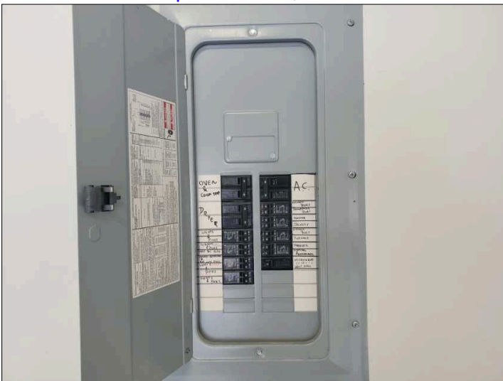
Panels that attach to exterior walls should be sealed on top and sides, but not bottom.
