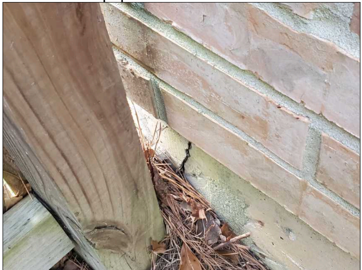
Corner pop noticed. Corner sections of the foundation are not supported as much as rest of foundation. This is not typically an issue, but take notice if cracks begin to form in bricks or mortar above corner pop.
