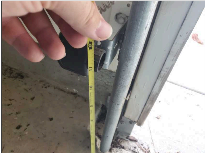
Opener sensing eyes higher than 6" above floor level.
