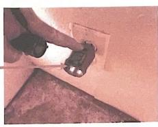
The outlets less than five and a half feet above the floor are not tamper resistant as required by today's standards.
