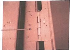
∑Damaged/decayed door was observed at the base of the door leading into the exterior storage area. Recommend repair/replacing.
