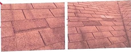
⊠Shingle granule loss exposing asphalt was observed.
