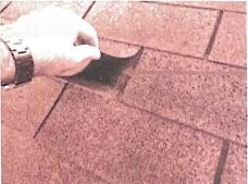
Multiple exposed nail heads were observed in some areas. Recommend sealing all exposed nail heads.
