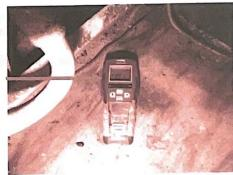
Existing/previous moisture penetration/staining were observed at the back right side of the attic however the inspector was unable to get to the area where the moisture penetration/staining was observed & could not determine if an active leak was observed. Recommend further evaluation.
