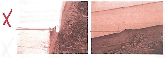
Deteriorated caulking/sealant was observed in some areas. Recommend sealing as needed.
